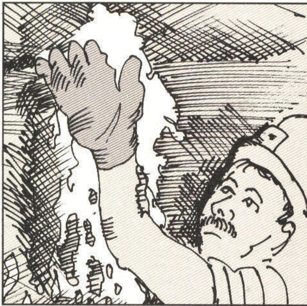
Application of AQUA PLUG to seal leaks
